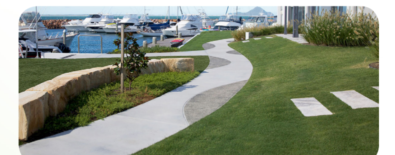
SHOTBLASTING CONCRETE TO FORM PATTERN
